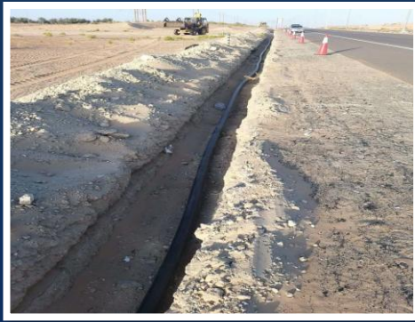
Fiber Cable Laying – Al Dafrah Laying of 8km of FOC for Al Dhafra Municipality 2022
